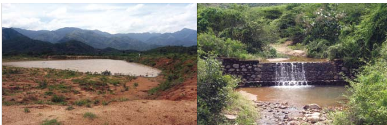
Check dams and other water harvest structures to control erosion are labour intensive to construct
